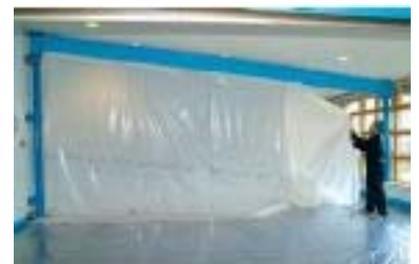
**After the construction work is complete we will technically clean any areas that require cleaning, provide air particulate readings to prove the room and work areas are safe, then remove the enclosure, handing the whole room back to the IT or Data Centre Manager.**
