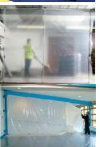
After the construction work is complete we will technically clean any areas that require cleaning, provide air particulate readings to prove the room and work areas are safe, then remove the enclosure, handing the whole room back to the IT or Data Centre Manager.
